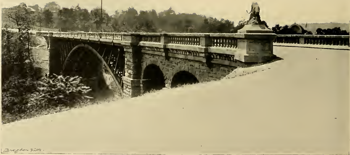
Bridge over Panther Hollow, Schenley Park.
